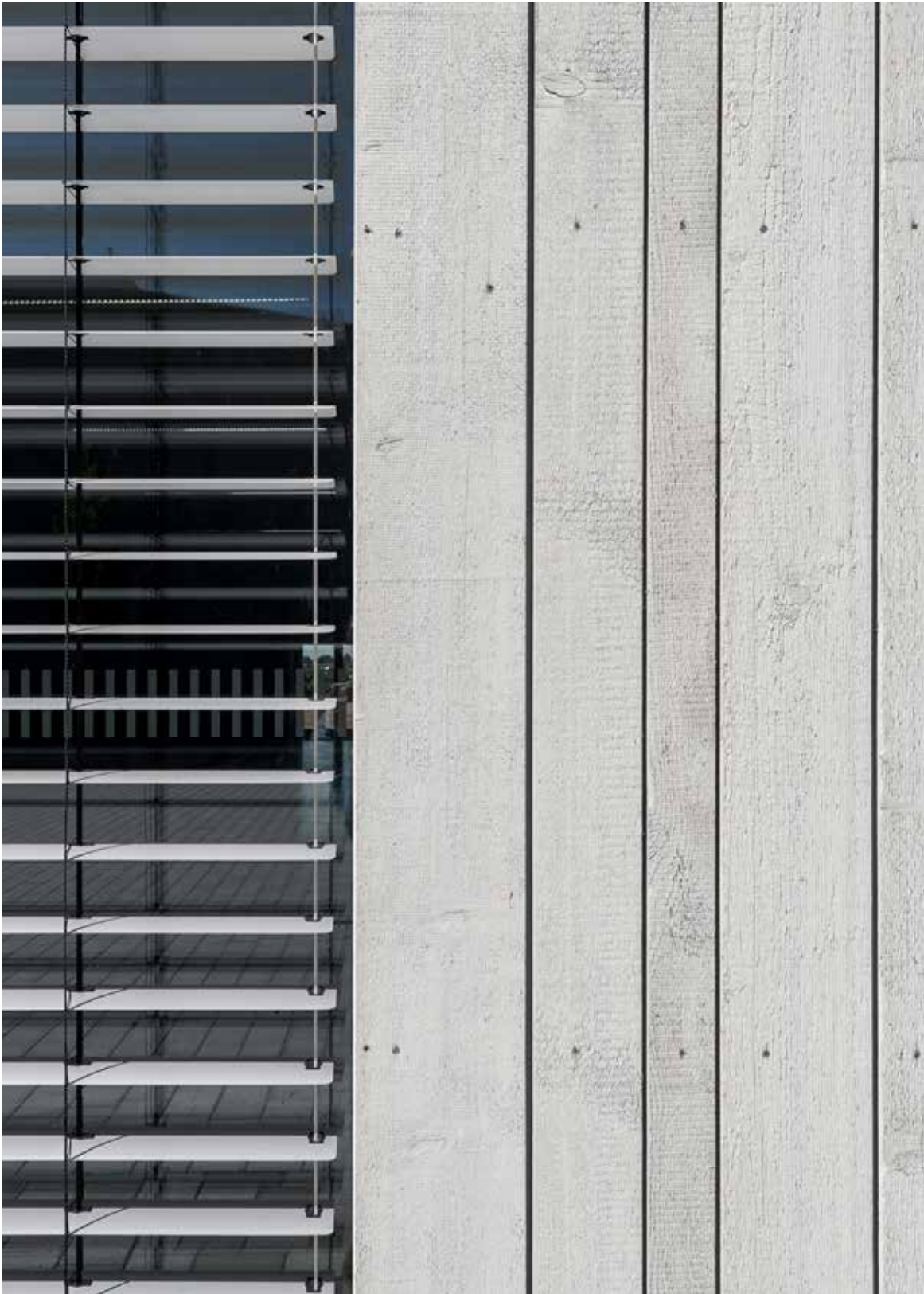
Glazed with KEIM Lignosil-Verano: The rough-sawn board formwork still shows a matt, open-pored surface.
